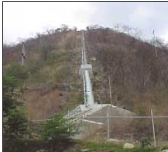
The penstock and powerhouse of the 13 MW Pasabien small hydro project.
